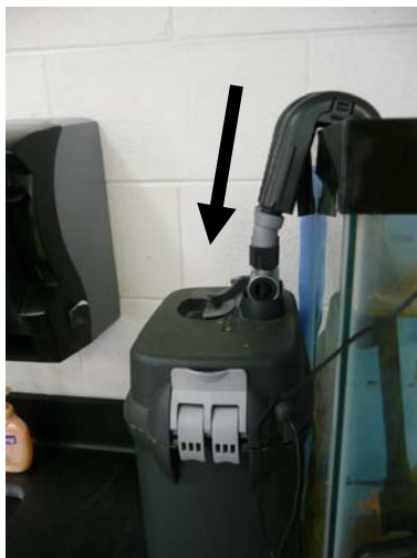
Tubes at too much of an angle
